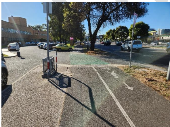
Figure 3.7 Inconsistent Line marking at the School Access and Shared Use Path
